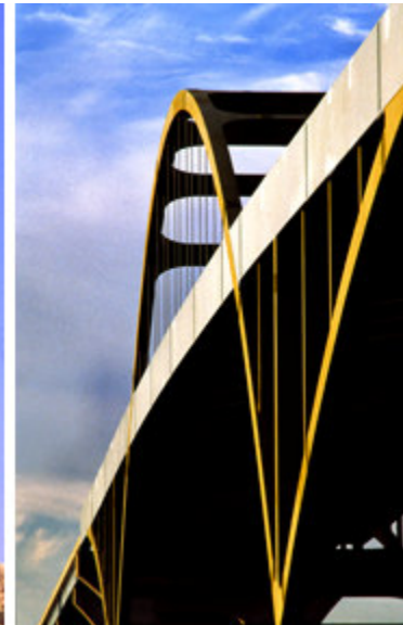
Milwaukee Bay Bridge
